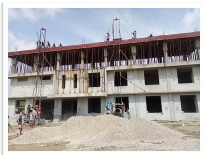
Eye Hospital under construction
