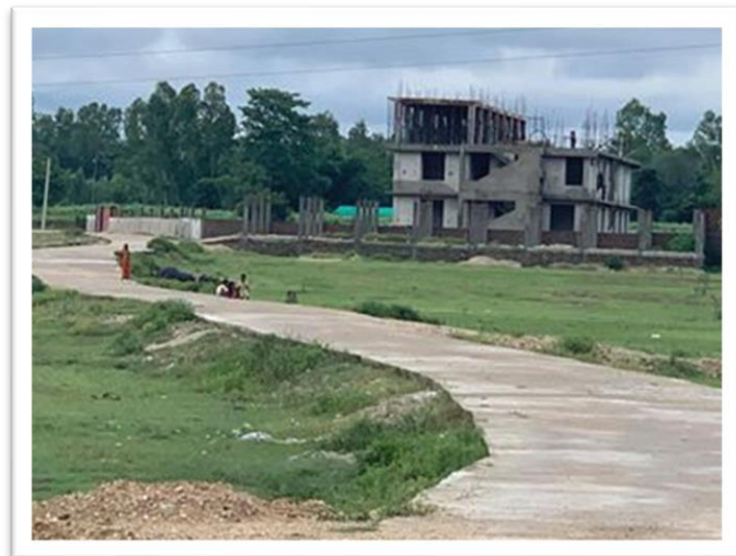
Access road to the new Eye Hospital
